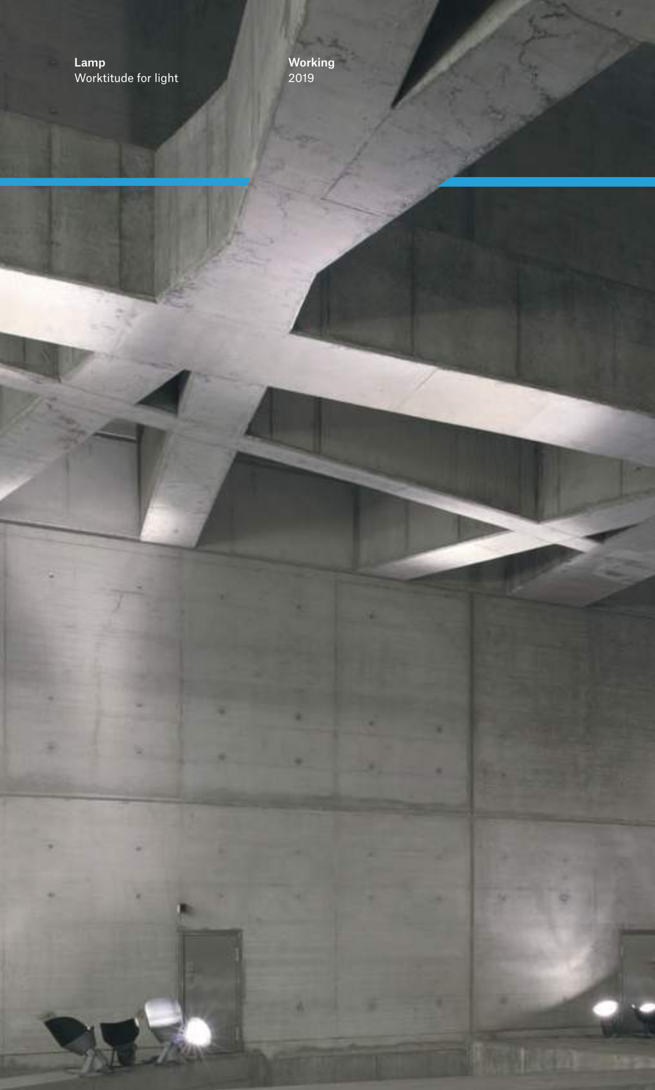
SHOT 290 Budapest Underground Line M4 - Kálvin tér Station, Budapest (Hungary)
